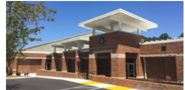
Chesterfield Administration Building
