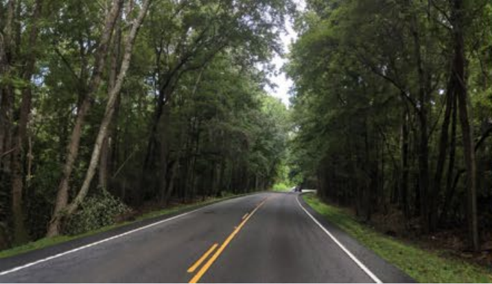
Rural Road Safety
